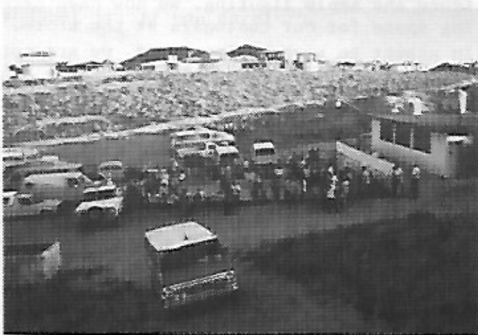
ROOF TOP VIEW OF THE NEW PATIO.
