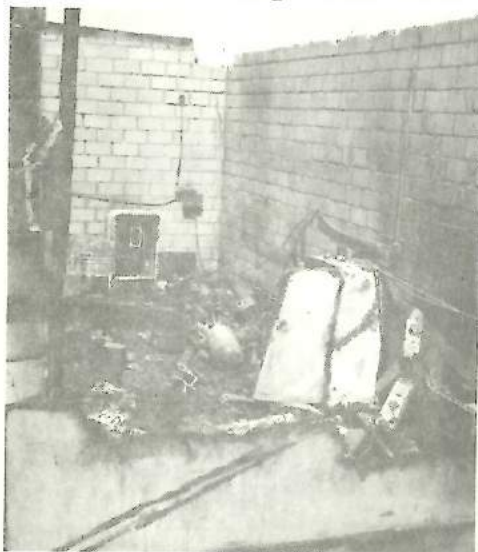
Remains of Walter Sheets' Cabin after the explosion
